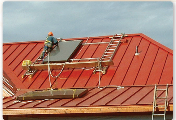
Solar hot water installation by a registered SolarBC installer.
